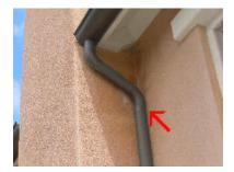
5. Need Attention, Installation of downspout extensions would help carry the water further away from the PLASTER SITE.
