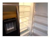
17. Attention Needed - There is a refrigerator installed. It appears that it does not level with floor and under the top cabinet, need adjustment.
