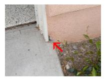
8. Need Attention, there is crack at the button of second floor balcony, that need touch up and paint.
