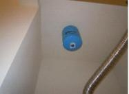
Safety Overflow Pipe: Satisfactory - The overflow pipe is correctly installed. Water Heater Insulation Jacket: No. Good - The visible portions of the hot water supply piping are insulated. This will Insulated Hot Water Piping: help deliver hot water to the faucets quicker with reduced heat loss. **Solar Assisted Water Heating:** None.
