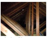
Roof Framing Condition: Roof Bracing: Satisfactory - The roof framing appears to be in functional condition. The roof framing as installed seems adequate.
